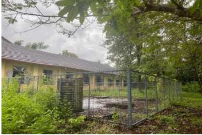
RAINWATER HARVESTING TANK
